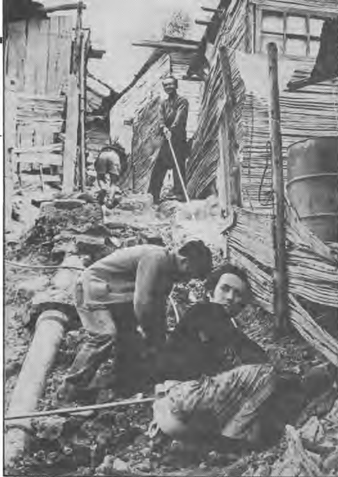
... installing water pipes by self-help groups in Colombia
